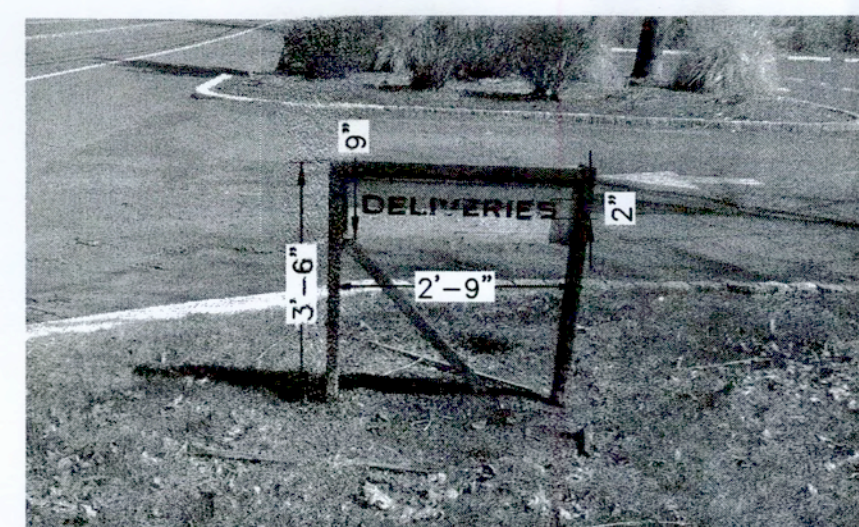
"ENTRANCE" & "DELIVERIES" SIGN DETAILS N.T.S.
